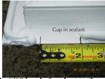
Apply 1/2" bead of sealant to the rear of the nail fin of the window, skipping (2) gaps on the lower nail fin. Set window in RO. Window must be level, square & plumb.
