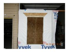
Cut house wrap as shown. Fold into RO at bottom and sides, Hold up at the top of the opening.
