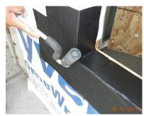
Cut two 9" squares of SAF and apply as end dams to the pan as shown. (One on each side.)
