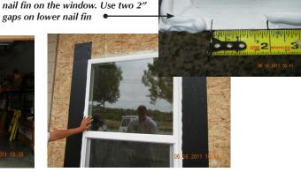
Apply 1/2" bead of sealant to the rear of the nail fin of the window, skipping (2) gaps on the lower nail fin. Set window in RO. Window must be level, square & plumb.
