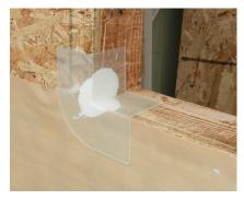
Apply sealant at the lower corners of the RO and set the Lightning Flash corners into the sealant as shown.
