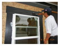
Apply the Top Flashing over the nail fin at the head of the window.
