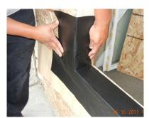
Cut two 9" squares of SAF and apply as end dams to the pan as shown. (One on each side.)
