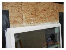
Apply screws every 12 - 18 inches. Wipe away excess sealant at the head of the window.
