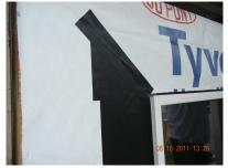
Apply the side flashing, install top flashing. Wipe away excess sealant at the head of the window before the top flashing is applied.
