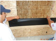
Hold the SAF water proof flashing membrane 3 inches over the framing sill and stick to the wall. Cut two vertical slices into the membrane as shown; lay the flashing on to the framing sill and remove all wrinkles.
