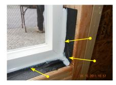
Apply sealant to the inside edge of the window as shown and tool into place.
