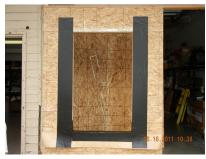
Apply side flashing as shown.
